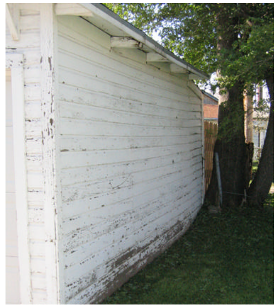
Garage, West Side
