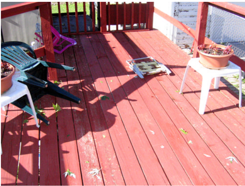
Deck floor and railing, speckled and dented from hail
