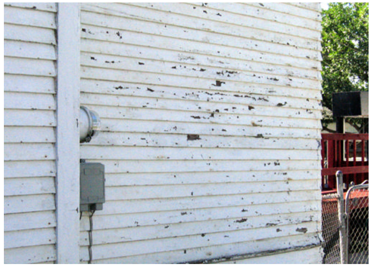
West, Rear of house
