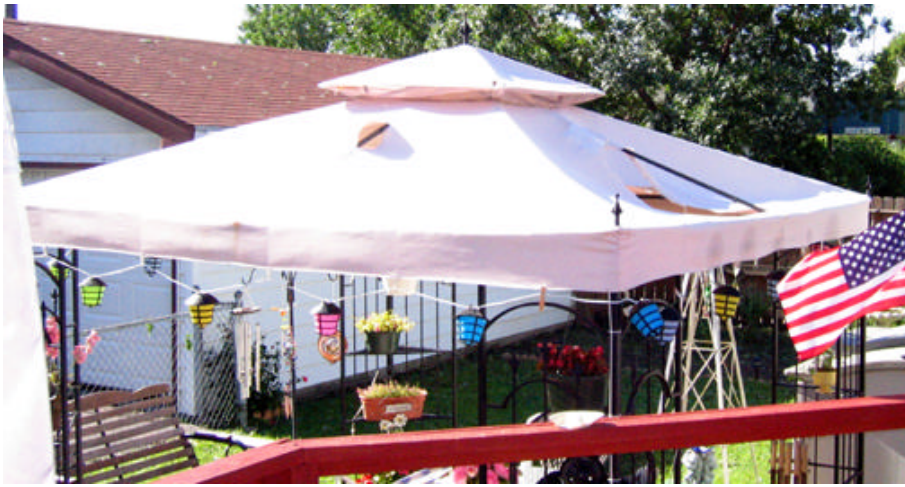
Gazebo Roof Damage
