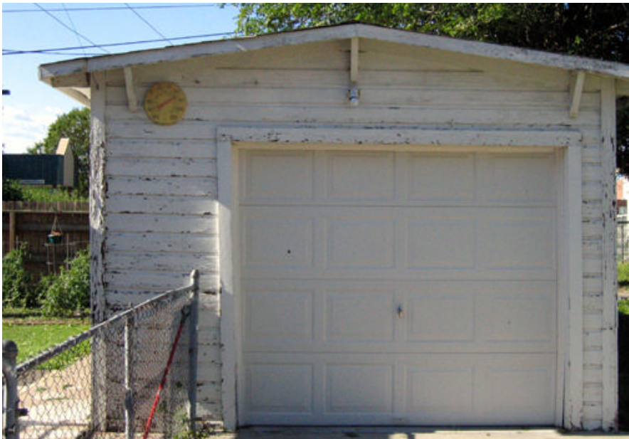
Garage North Side
