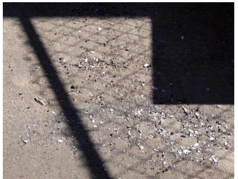
Roof Gravel and house paint from downspout
