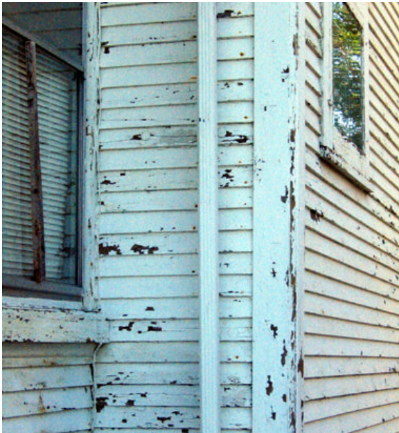
Front, West Corner of House
