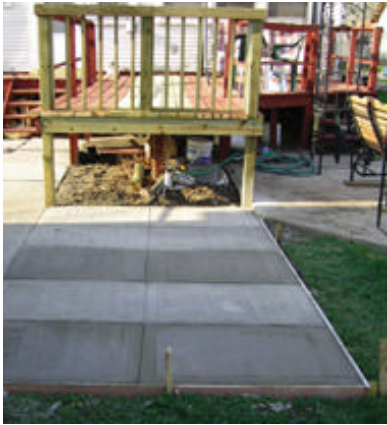
Sliding gate is installed
