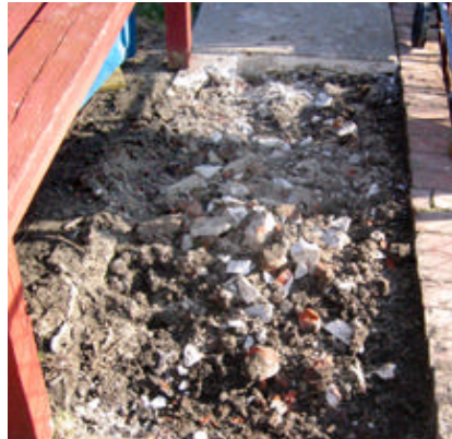
Two sections of sidewalk had to be broken, removed and replaced with new concrete (right), making it more negotiable for the scooters.
